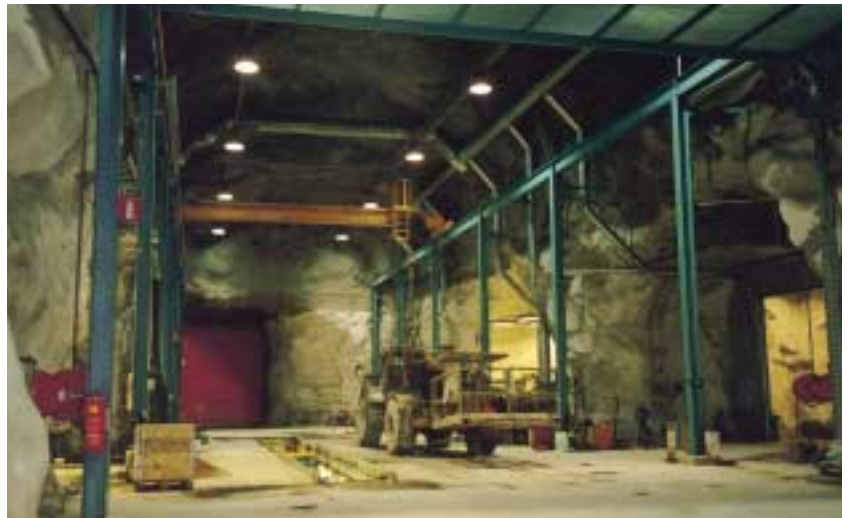
Inside the 350 m-level workshop at Kemi.
