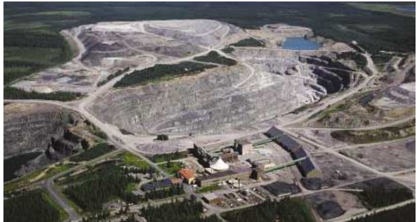
Aerial view of Kemi mine, located close to Finland's border with Sweden.
