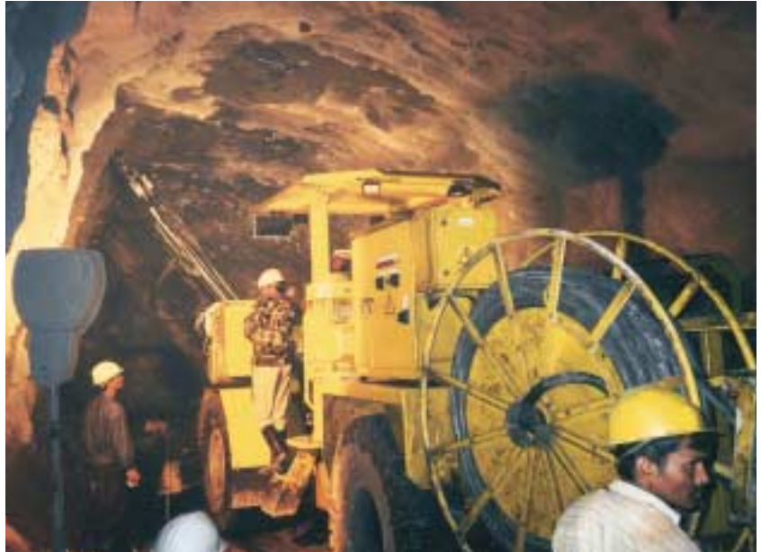
Atlas Copco Rocket Boomer 352 at junction of Mirchingchu Adit with HRT.
