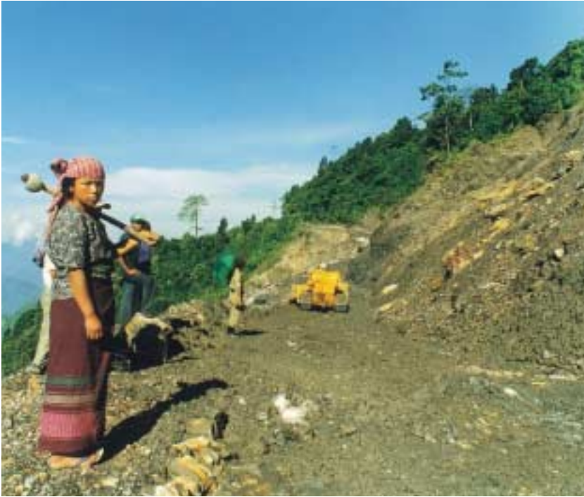
Repairs underway on Bhutan National Highway No 2.
