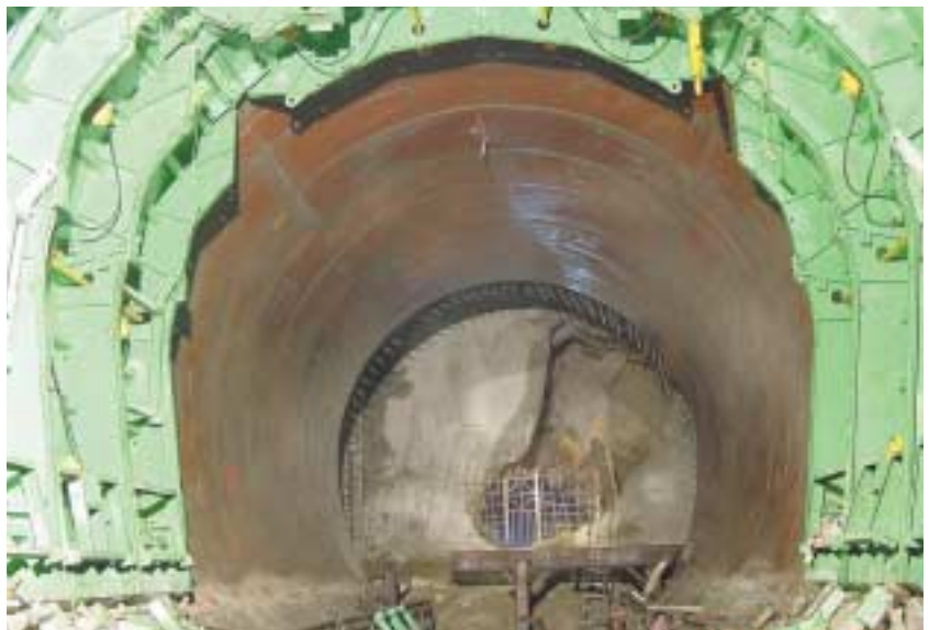
Lining the head race tunnel at Tala Hydro.
