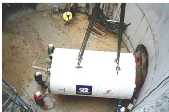
Picture 1: The Lovat TBM at the bottom of the launch shaft.
