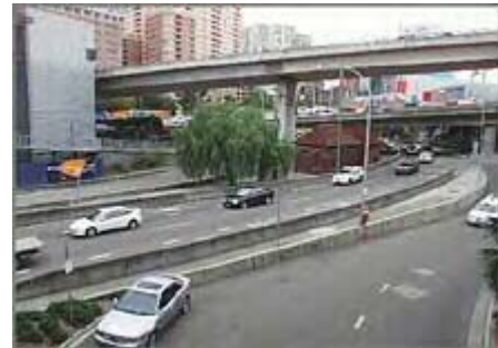
Picture 1: The site where the Cross-City tunnel will join the Western Distributor.
