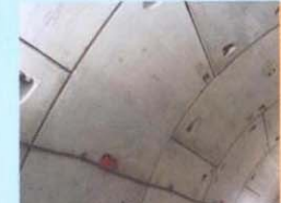
Picture 3 (left): The concrete segments are equipped with yellow ring connectors on their back edge which are plugged to the previously installed ring and blue connectors on the front edge to which the next ring will be connected.
