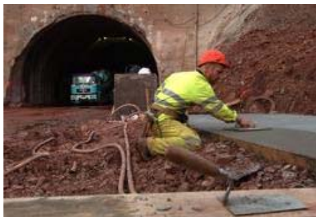
Picture 1: The 610 m-long 9 m-wide Schirmeck tunnel (Rothau side).
