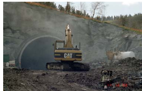
Picture 1: Portal of the San Marcial tunnel.
