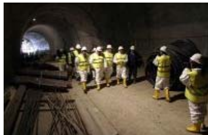
Picture 1: Visit of the Ibaeta-Amara tunnel after breakthrough.
