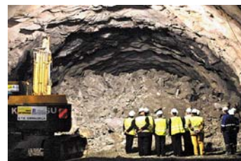
Picture 1: Breakthrough of the Gibralmora tunnel.
