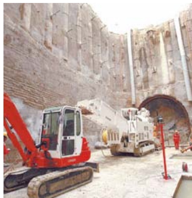
Picture 2: Sébeillon start box for the tunnel drive towards the Tridel plant in La Sallaz.
