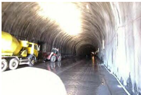
Picture 1: The Varen tunnel on 15 th July, 2002.
