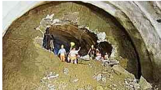
Picture 1: Holing through of the Monguelfo bypass tunnel.
