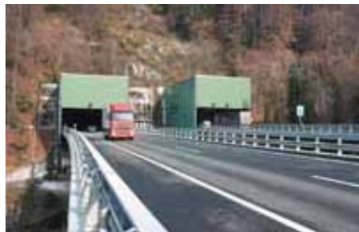
Picture 3: Portals of the Glion tunnels.
