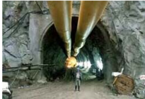
Picture 1: Headrace tunnel of Tala hydro scheme.
