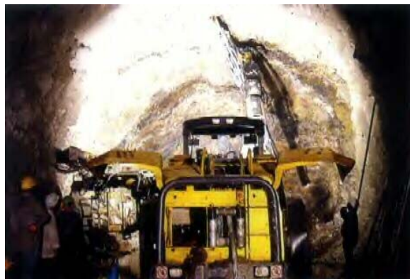
Picture 2: Rock bolting at Kalikhola Downstream.
