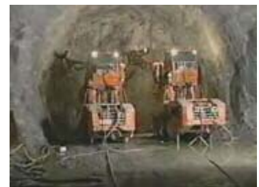
Picture 1: Tamrock Axera T12 jumbos working at Toulousteouc.
