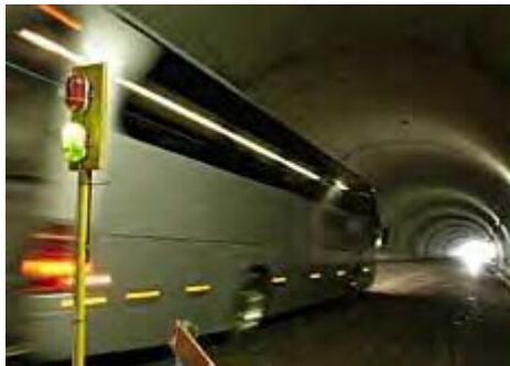
Picture 4: The third Baregg tunnel will help ease congestion on the Bern to Zurich motorway.
