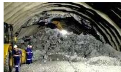
Picture 3: Last blast at the Tevilla tunnel.
