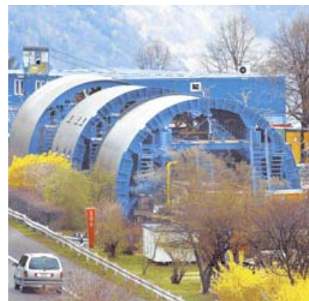
Picture 2: Formwork units at the Glion tunnel.
