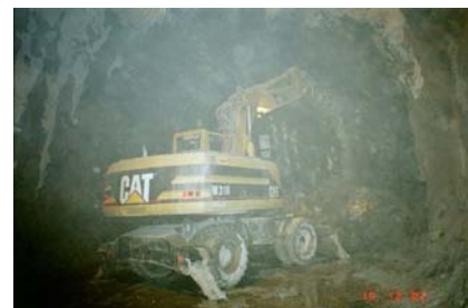
Picture 3: Work on the Geriátrico tunnel.
