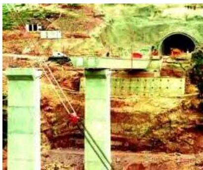
Picture 2: The La Riba (Alt Camp) tunnel and viaduct.
